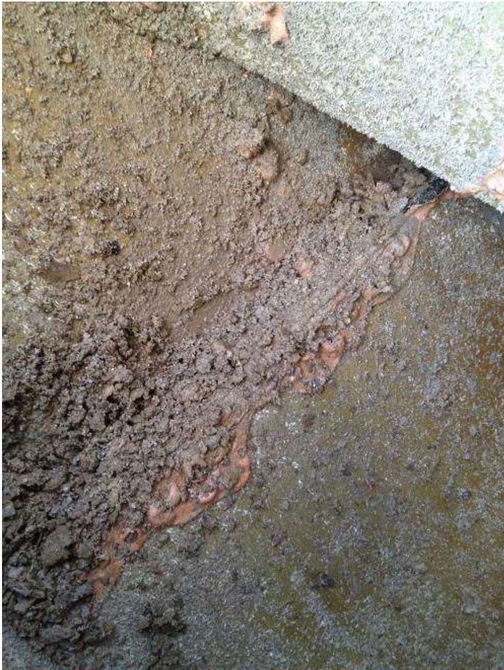
CT2 – Prior to work commencement.
