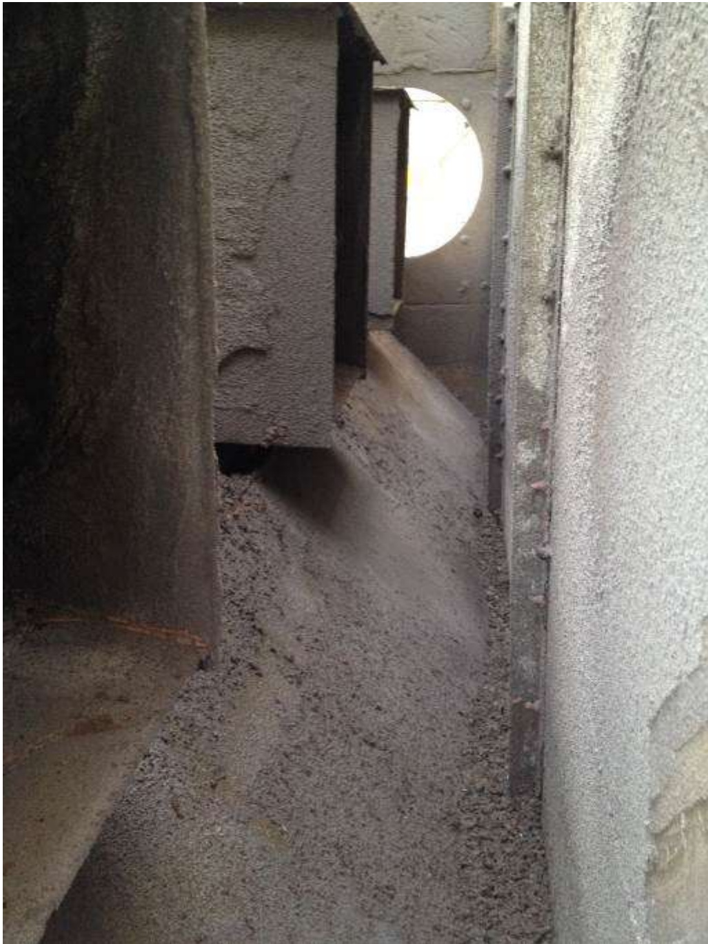
CT2 – Prior to work commencement.
