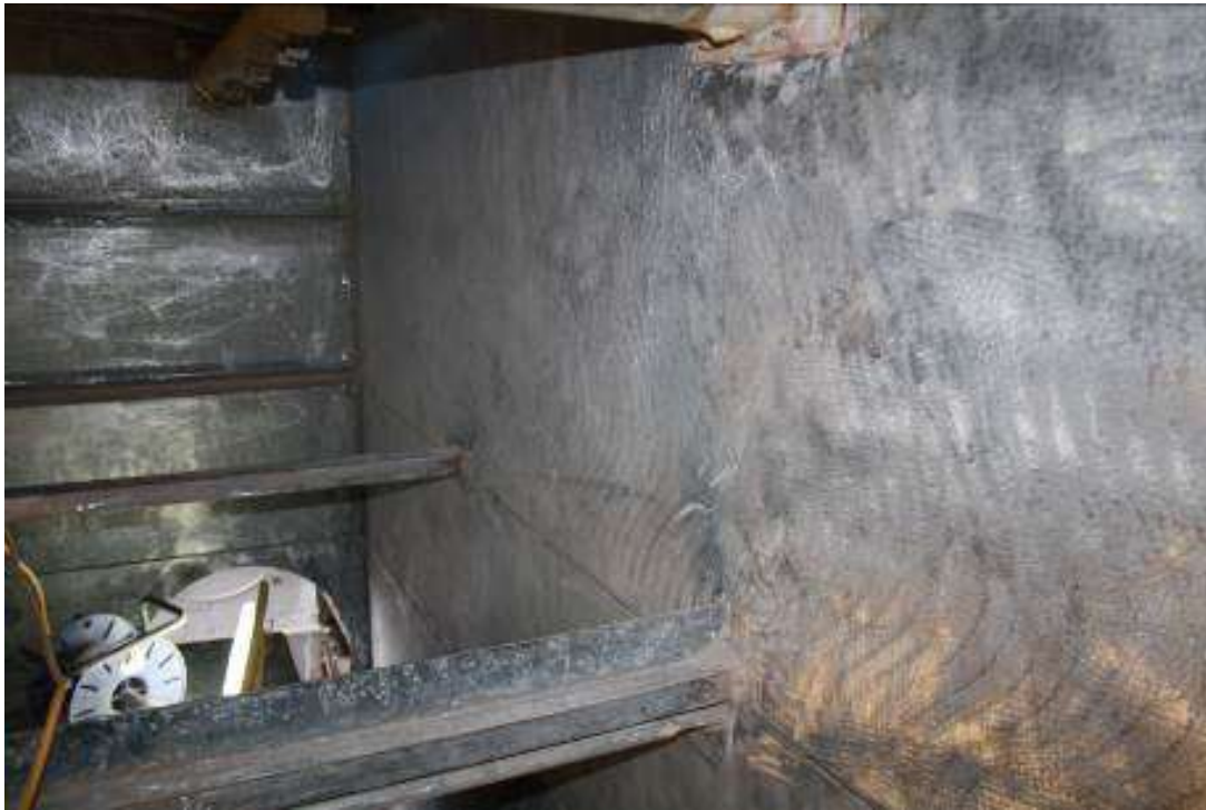
CT2 –Surface preparation
