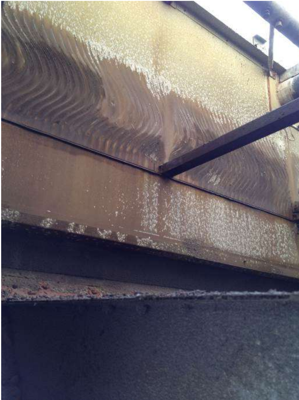
CT2 – Prior to work commencement.
