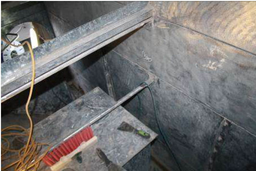
CT2 –Surface preparation
