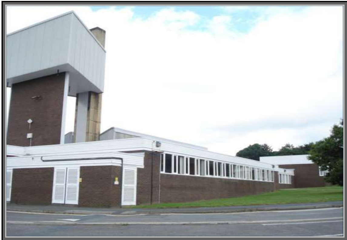
External picture of Tank Tower (20m high from ground level)
