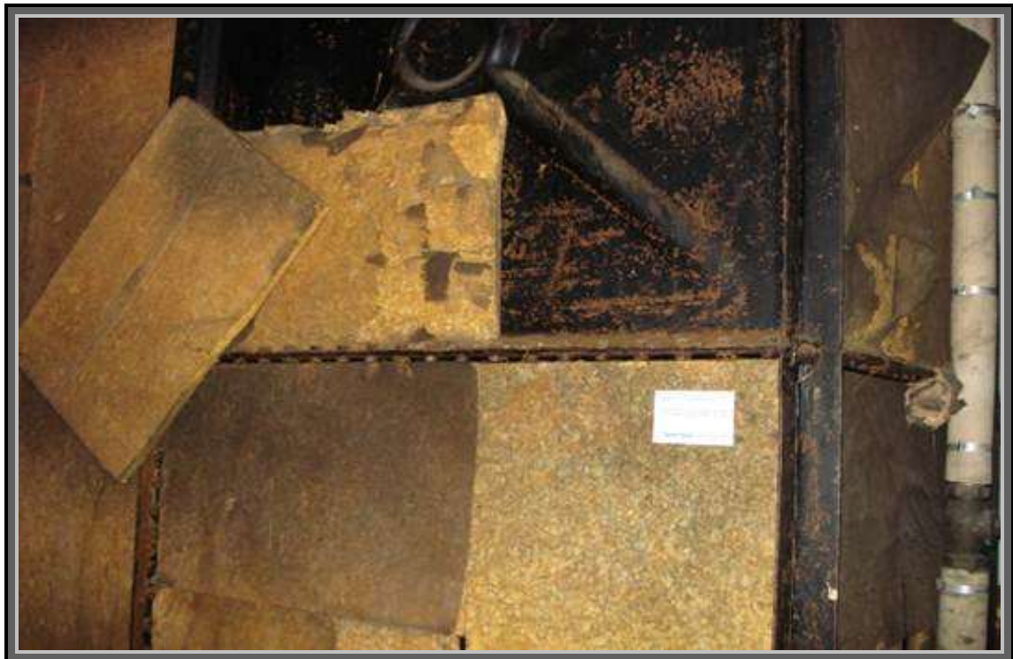
External picture of CWST within the Tank Tower
