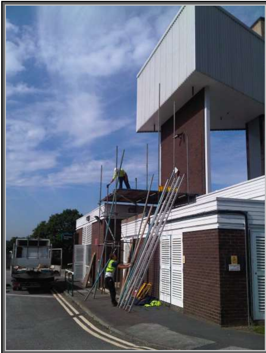
Scaffolding been erected (day 1)
