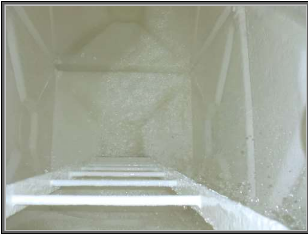
Water tank re-filling & been returned to service
