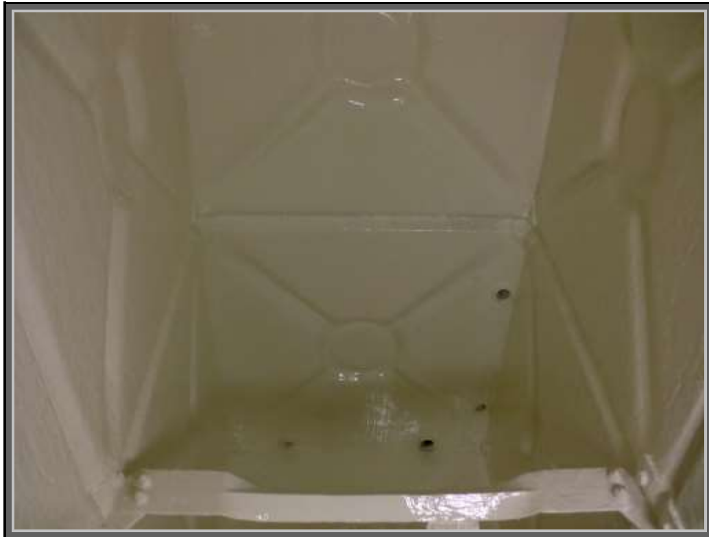
Anti-corrosion treatment completed
