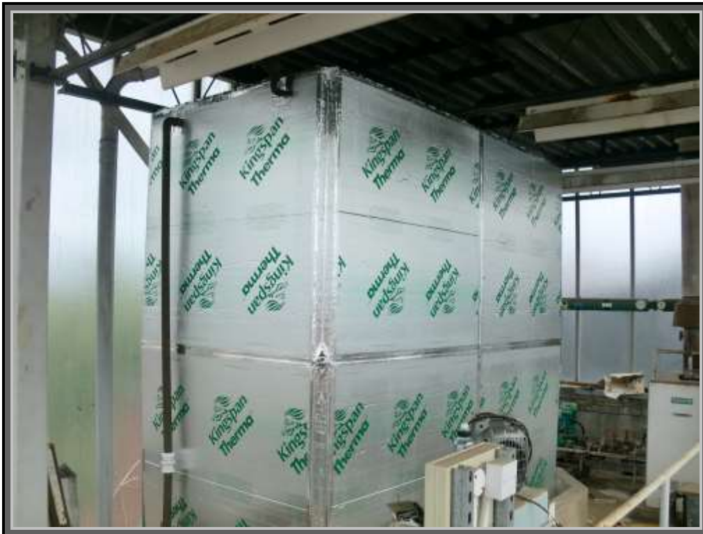
External picture upon completion of the works to CWST 1
