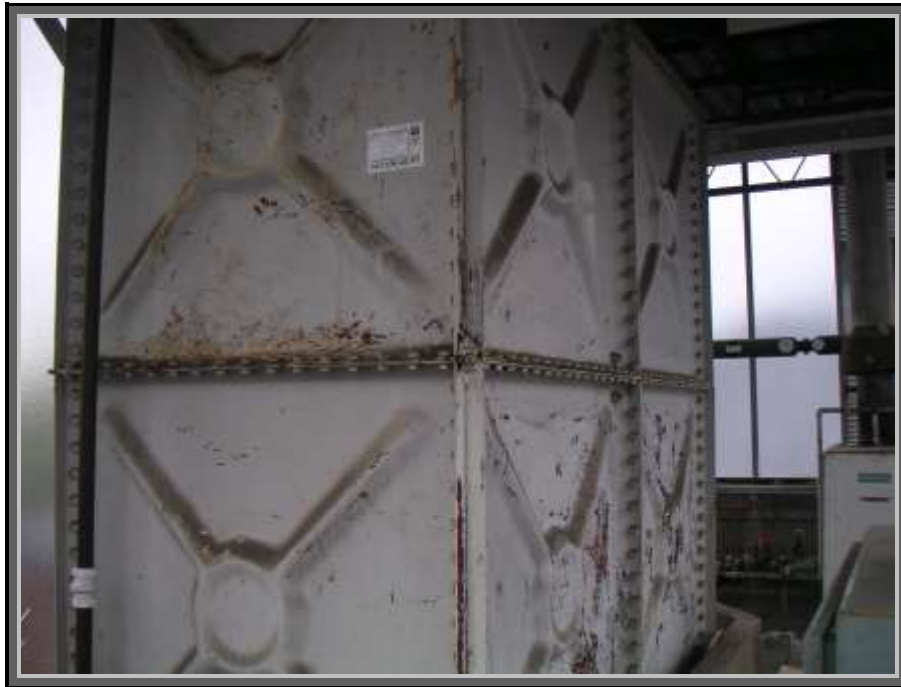
External picture of CWST 1 before the commencement of works
