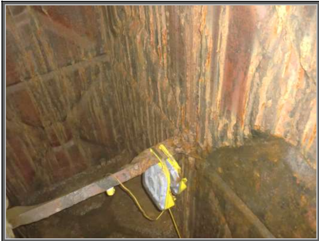
Internal corrosion
