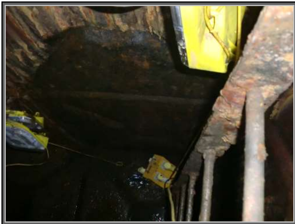
Internal corrosion
